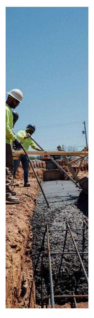
consist of 5 men on a crew. 1 footer foreman, 1 layout foreman, and 3 concrete mechanics. ECI has 2 full fledged footer crews. Our footer crews go to all job sites that require footers and poured walls. The footer crews show up and pre-tie all the rebar needed to be installed in new excavated footer trenching and poured walls also. Lay out
